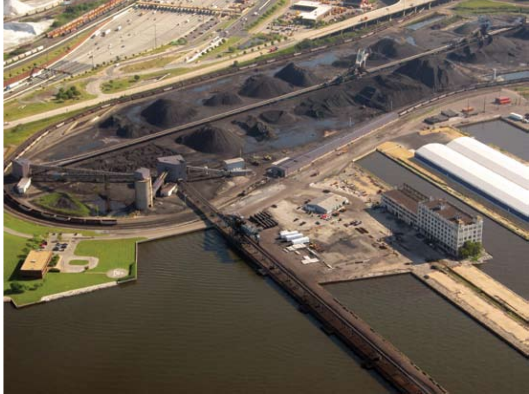
Coal burned in power plants—such as these piles of coal outside a Baltimore power plant—creates solid residues that often are disposed of in landfills. Credit: Joanna Woerner, IAN UMCES ( ian.umces.edu/imagelibrary )
