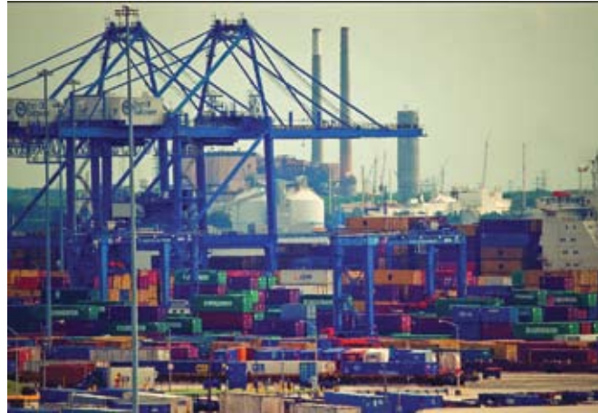
With its extensive facilities, the Port of Baltimore could become part of a competitive manufacturing hub for offshore wind components. Credit: Richard S. Quarles Sr., Voxefx Photography, www.voxefx.com
