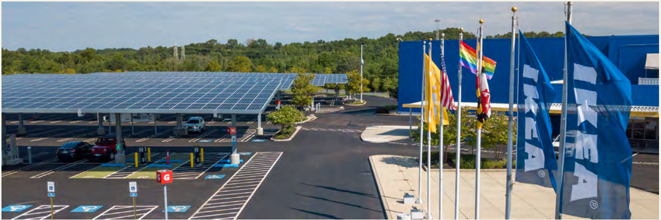
Solar parking canopy at IKEA Baltimore. Photo credit: IKEA
